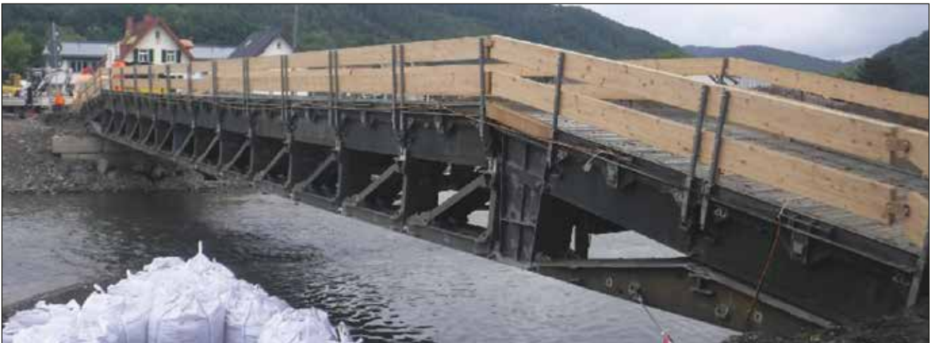
Abbildung 5: K 25 – Ahrbrücke Insul, Medium Girder Bridge der Bundeswehr, August 2021
